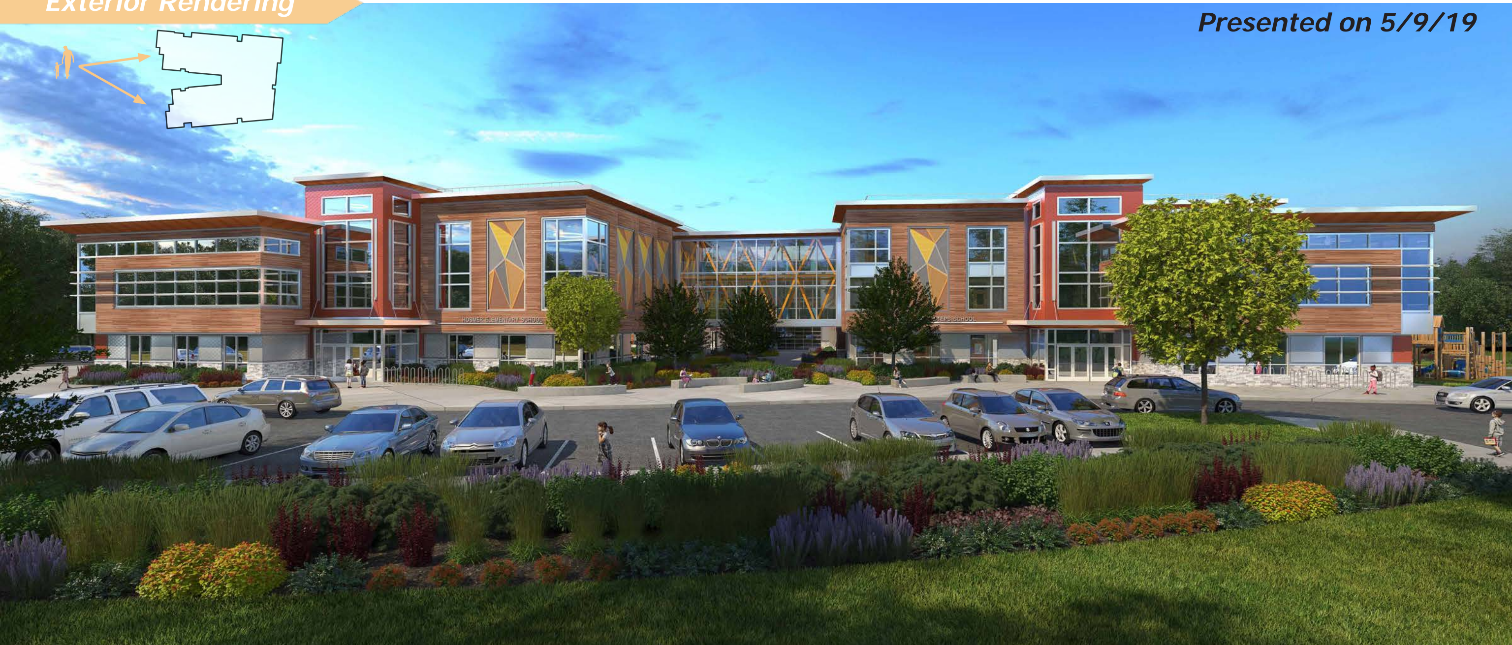
View of the east facade, showing main entries
